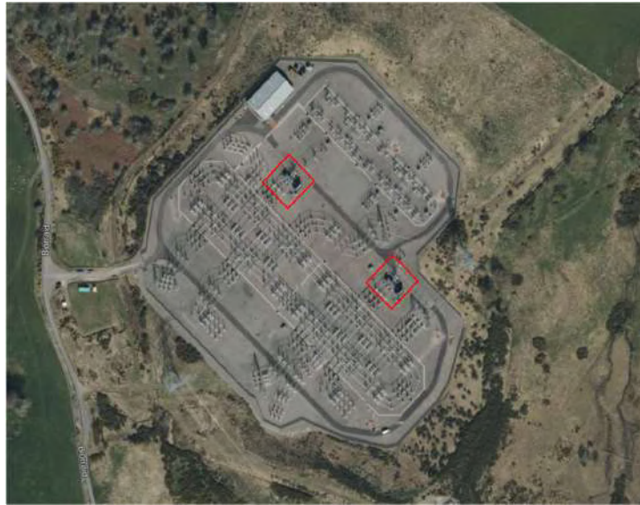
Figure 1 – Knocknagael Substation, with Transformers Highlighted
