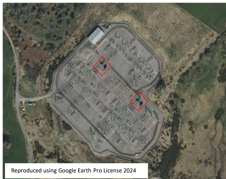
Figure 7-1: Knocknagael 132 kV Substation, with Transformers Highlighted
